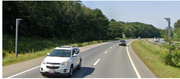
Overheight Vehicle Detection System on I-295 in Brunswick, ME
