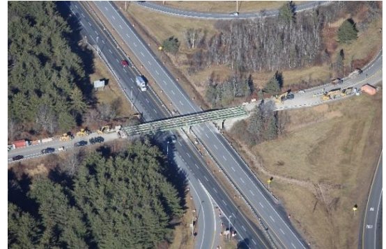
I-95 Exit 109 Ramp F Bridge Damage
